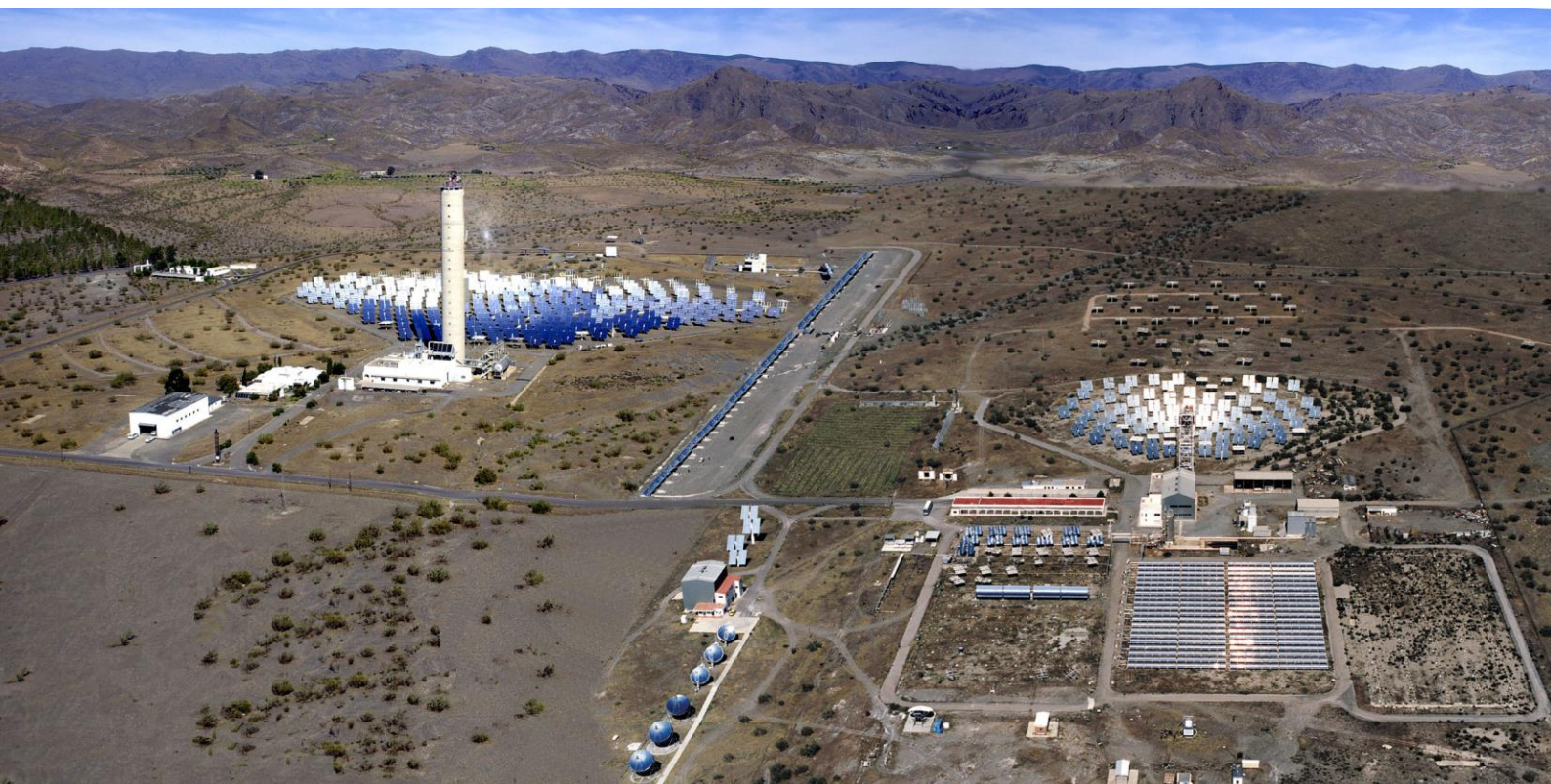
Figure 1. Aerial view of Plataforma Solar de Almería (PSA)
