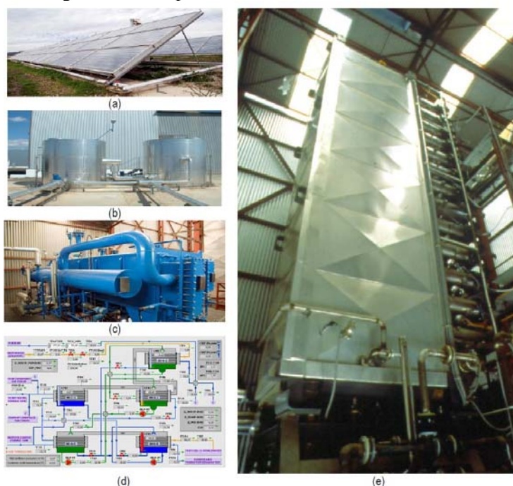
Figure 4. AQUASOL Solar desalination plant: (a) Solar field, (b) storage tanks and building of the solar desalination plant at PSA and (c) double effect heat pump (d) SCADA of the DEHP (e) MED desalination plant.
