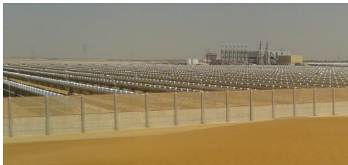
Figure 11. Typical wind and sand barrier erected in SHAMs (UAE)
