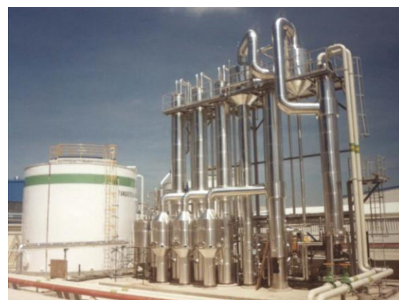
Figure 20. MEE plant installed in El Sauz (Mexico) MEE is coupled to a Combined Cycle Gas Turbine
