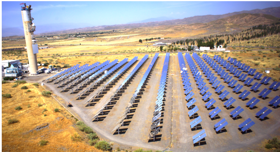
(b) CESA-I STP plant
